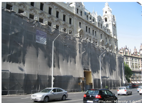
Figure 5: Scaffold covered by raschel net
