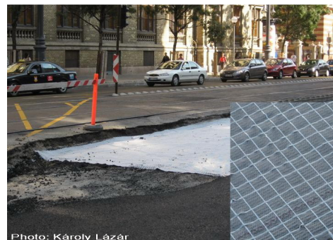
Figure 6: Knitted composite fabric used for driveway reinforcement
